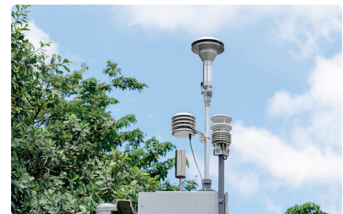
Figure 7.5: Smart Air-quality Station
